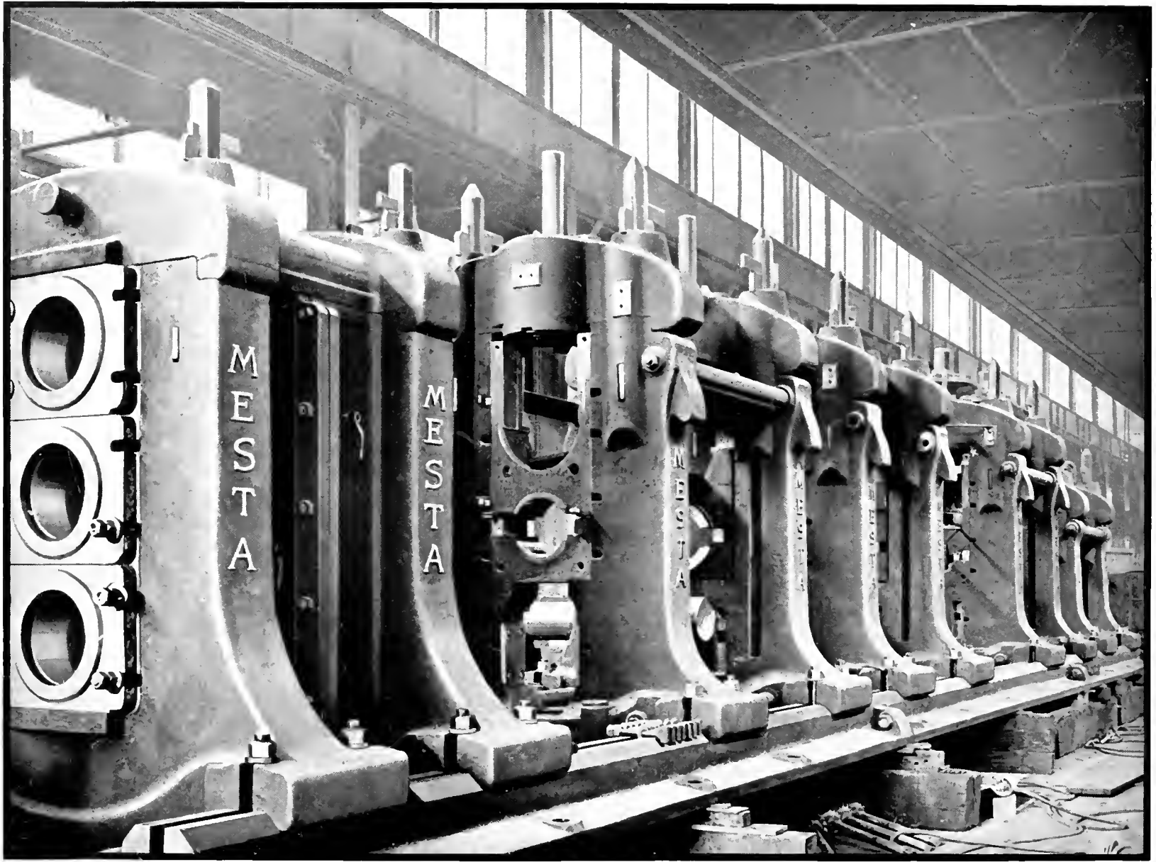
Bar Mill on Erecting Floor
